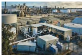
Torrance Refinery Water Recycling Plant Torrance, CA 6 MGD
