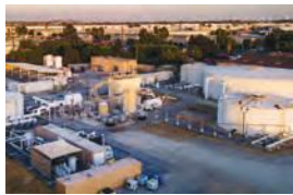
Juanita Millender-McDonald Carson Regional Water Recycling Plant Carson, CA 3-4 MGD
